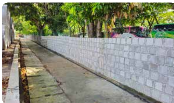
Perimeter fencing in HCCT Kuantan constructed with used concrete cubes
