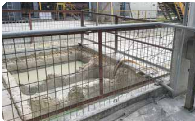
Slurry pits located at the Hume Concrete Beranang plant
