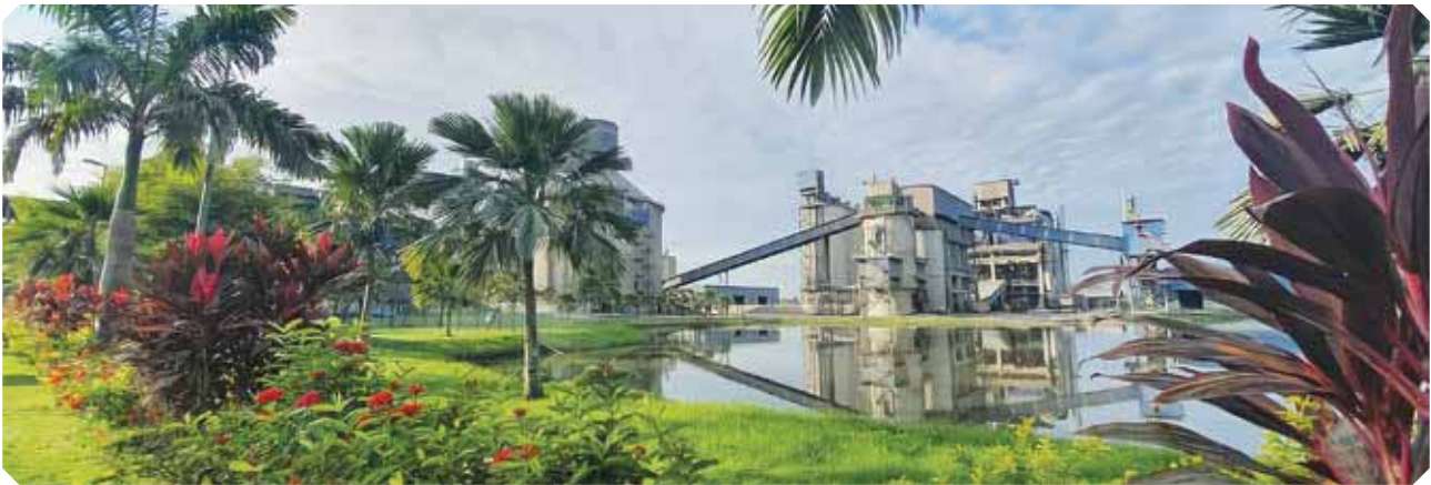
Retention pond located at the Hume Cement plant in Gopeng
